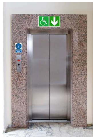
Designation example of an evacuation lift Foto: © Schwarz Brandschutz
